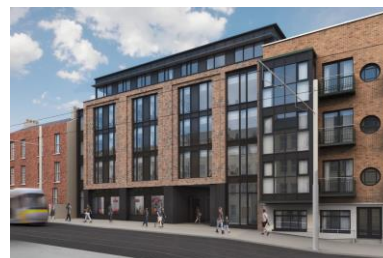
Dominick Place, Dublin, 320 beds, expected opening September 2019
